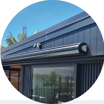
FACE FIX INSTALLATION
