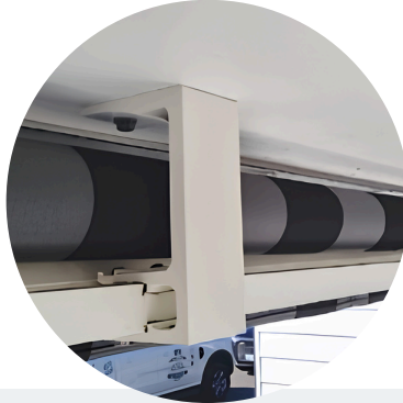
UNDER SOFFIT INSTALLATION
