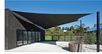
No fabric is cut until our poles are installed and the sail measurements checked to ensure 100% accuracy in fit and tolerance.
